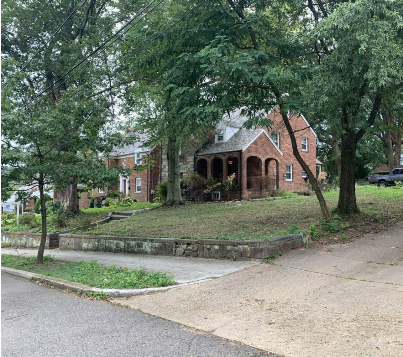
SITE FROM SIDE ALLEY WAY
